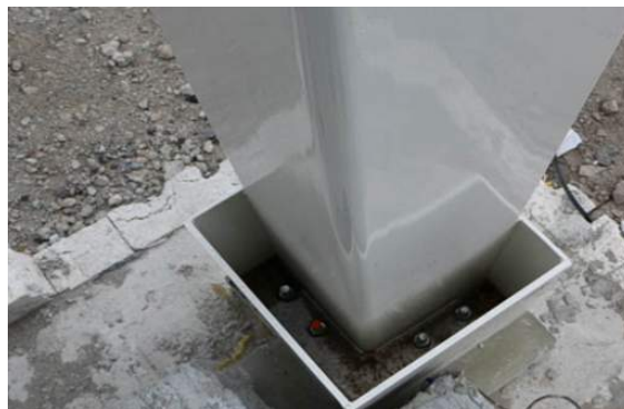
Figure 4. Demountable Connections in Fokker 7/8 Distribution Center, Schiphol Airport, the Netherlands
